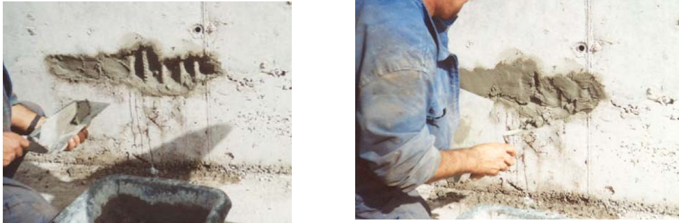
Photograph 1.- Placing of MAXREST ®
