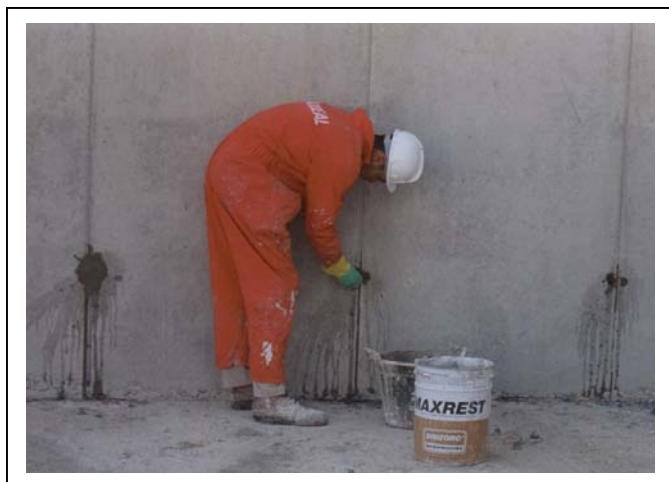
Figure 10. Treatment for opening on concrete surface.
