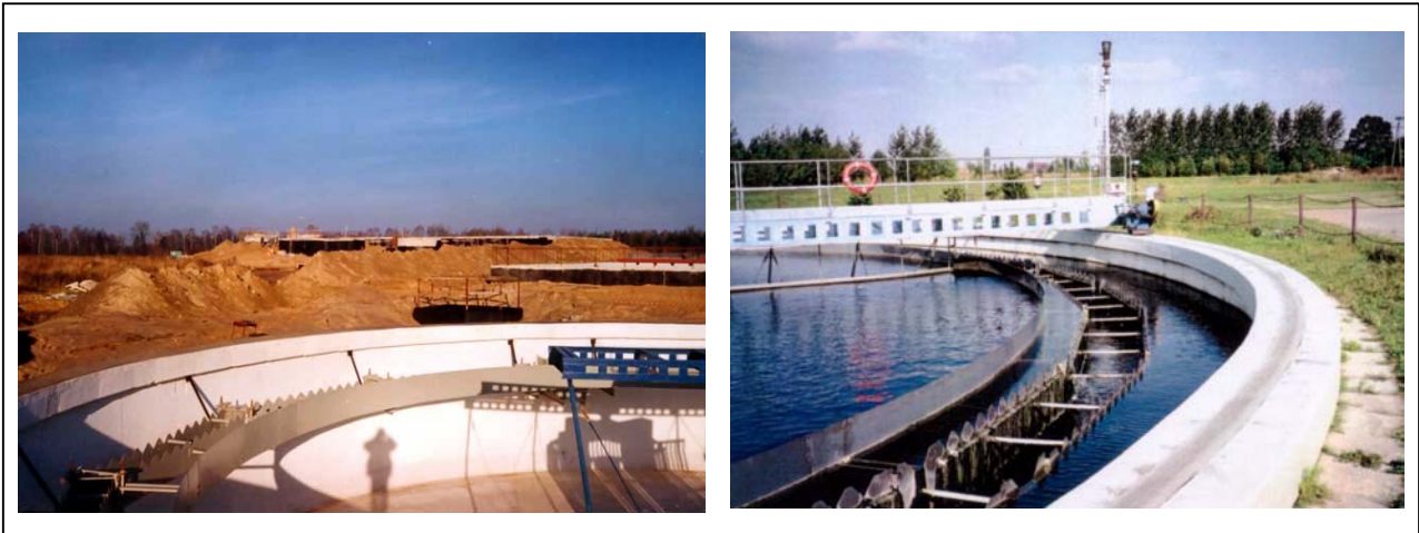
Figure 14.- Application of MAXSEAL®-/FLEX in primary/secondary clarifiers.
