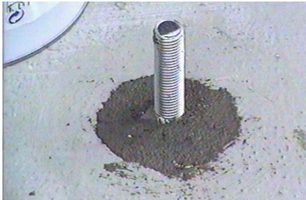
Figure 27.- Anchoring on horizontal surfaces with MAXGRIP ® and MAXGROUT ®
