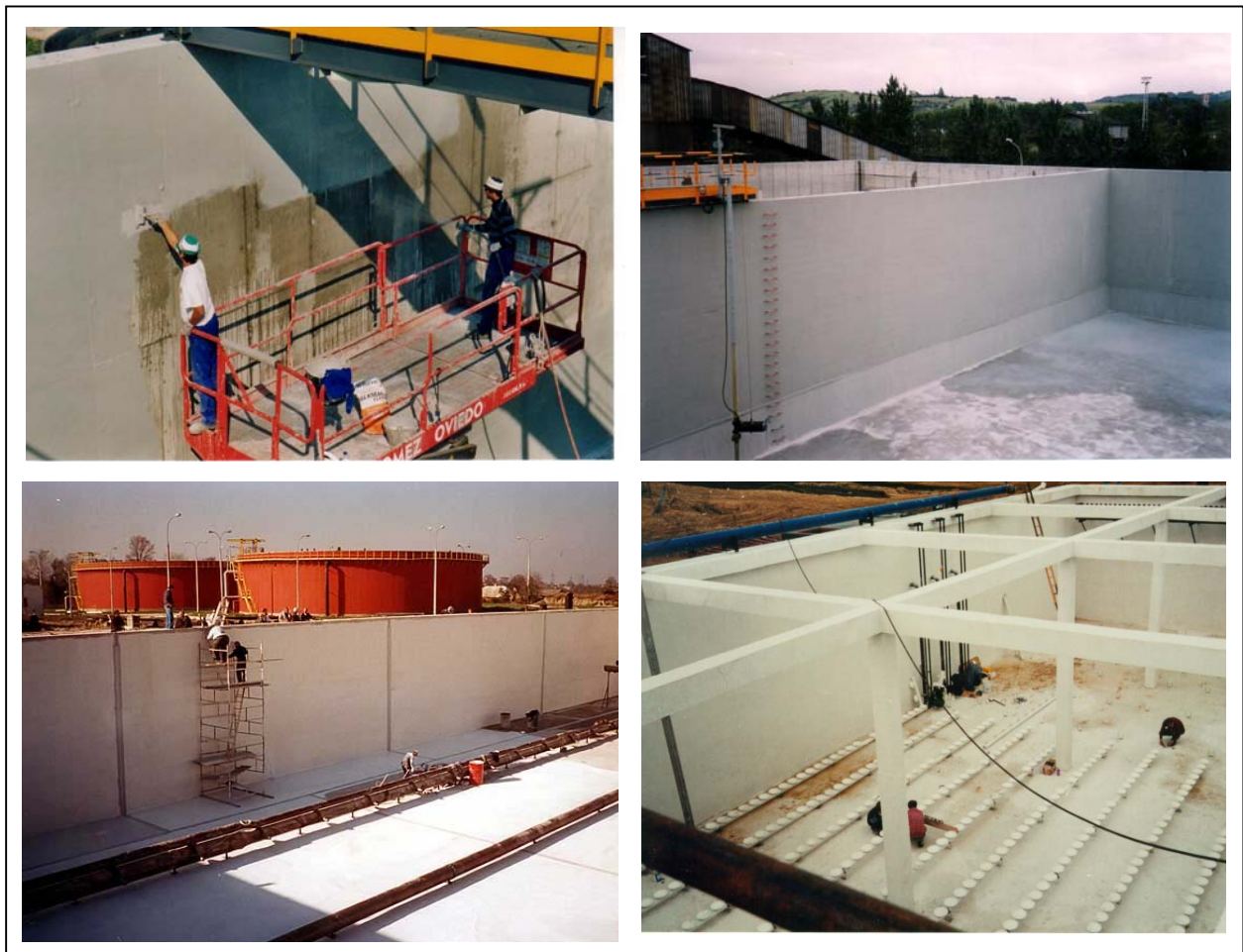
Figure 13.- Application of MAXSEAL® -/FLEX in aeration tanks.
