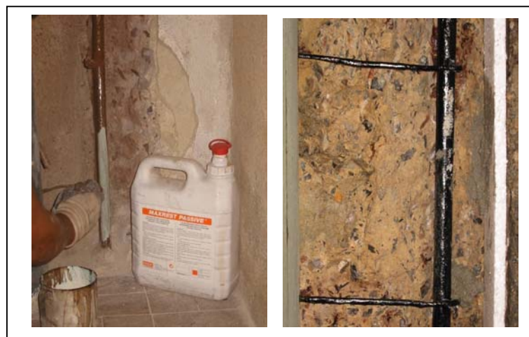
Figure 29.- Passivation of reinforcements with MAXREST® PASSIVE ,
