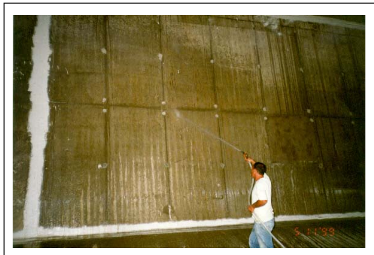
Figure 12.- Washing down the surface to be coated with MAXSEAL® -/FLEX
